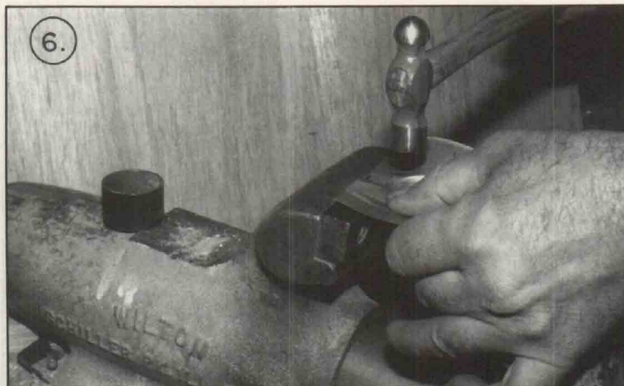
Straighten the flange edges a bit, any way you can. Use a small hammer and a steel back-up block (bucking bar), squeeze the flange edges in a vise, or simply hammer them flat.
